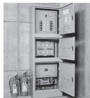
Distribution boards for construction work
